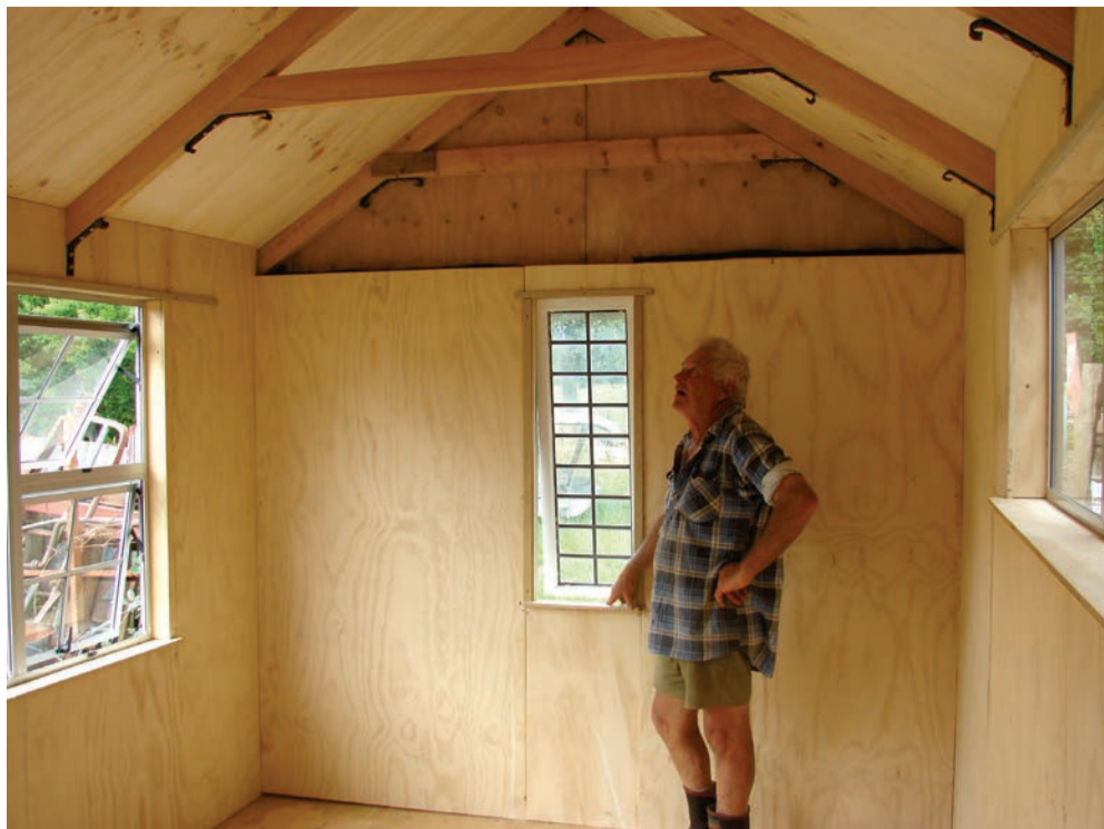
Nearing completion Malcolm inspects his latest building under construction. The gables inside are both attractive and make for extra strength. Low maintenance aluminium joinery is another important feature. This one will be finished with interior staining, as well as having an appealing veranda.
